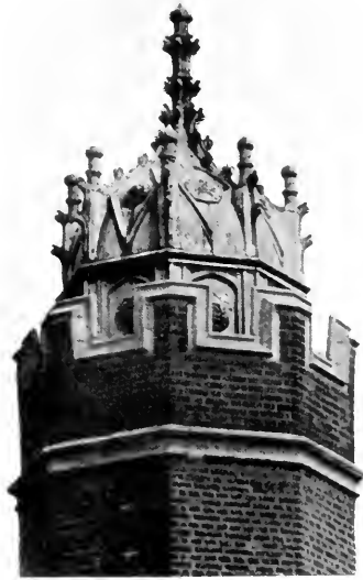
110. Lead Cupola, Hampton Court.
